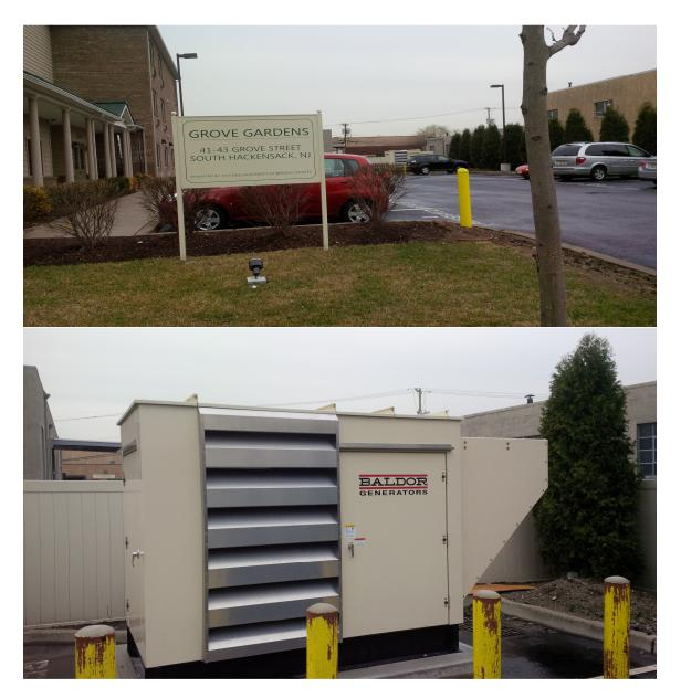
Installation of a new 100kW, 3-Phase Standby Natural Gas Generator at "**Grove Gardens**", residential housing complex operated by Housing Authority of Bergen County, NJ. The project consisted of new emergency power distribution system and natural gas plumbing design to provide emergency power to all house loads, including the elevators and kitchen equipment.
